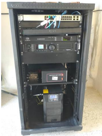
Fig. 5. - Equipment used at the company's infrastructure sites [1]
